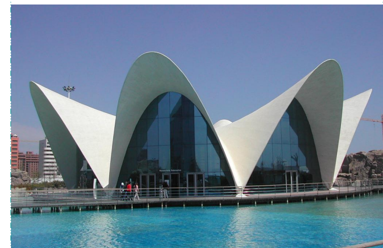
Steel fiber reinforced concrete thin shell structure Oceanographic Park Restaurant. City of Arts and Sciences , Valencia (2002) Based on blueprint of Felix Candela, by: A. Domingo, C. Lázaro, P. Serna
